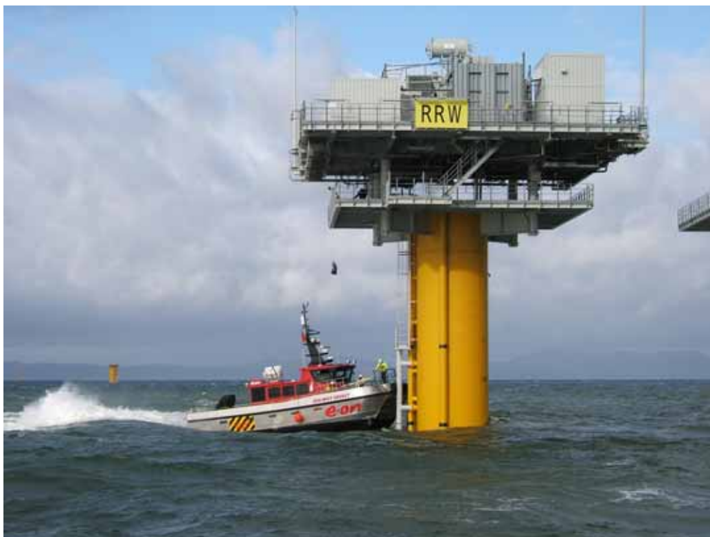
Figure 2.4: Photograph of an offshore substation at Robin Rigg Offshore Wind Farm
