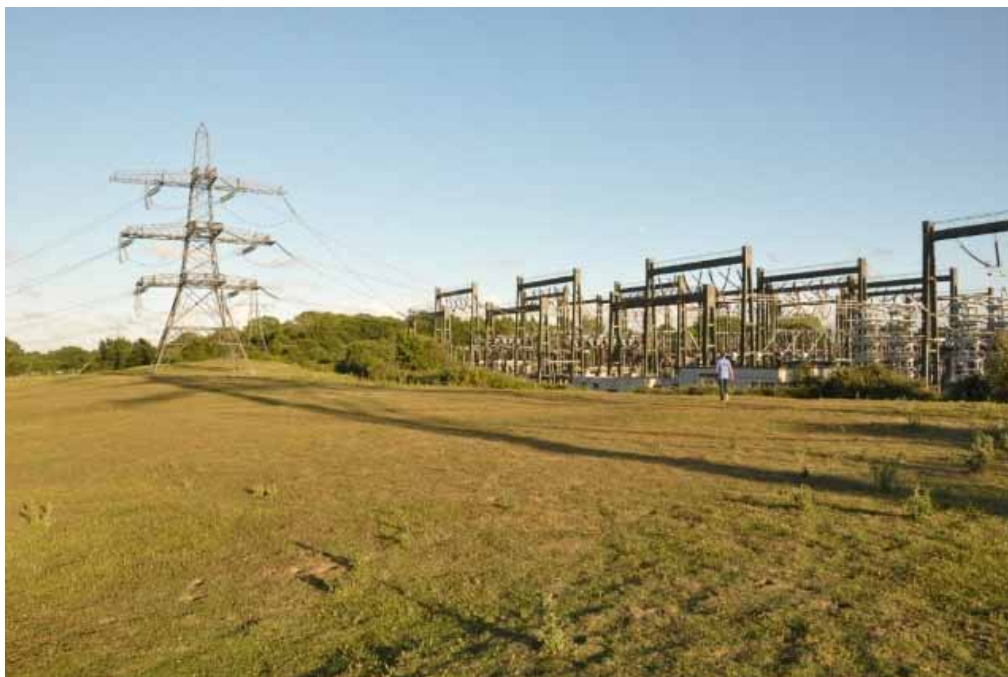
Figure 2.5: Photograph showing the existing Bolney substation site
